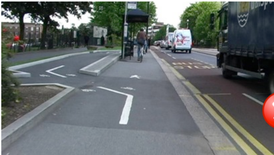
This cycle lane, directly outside the Town Hall, Forest Road, turns sharply around a bus stop - a difficult manoeuvre for novice cyclists. Lanes that veer suddenly, particularly onto or off roads, are not good design.
