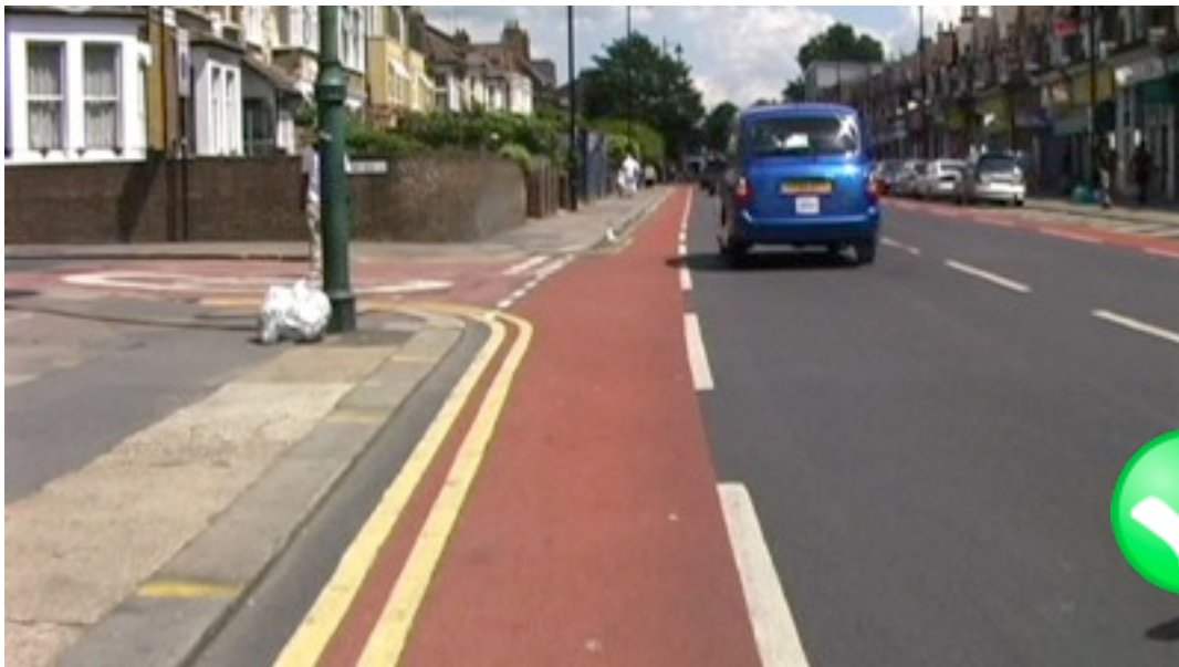
A reasonably wide lane that clearly has priority over the side road, encouraging drivers to think before turning.
