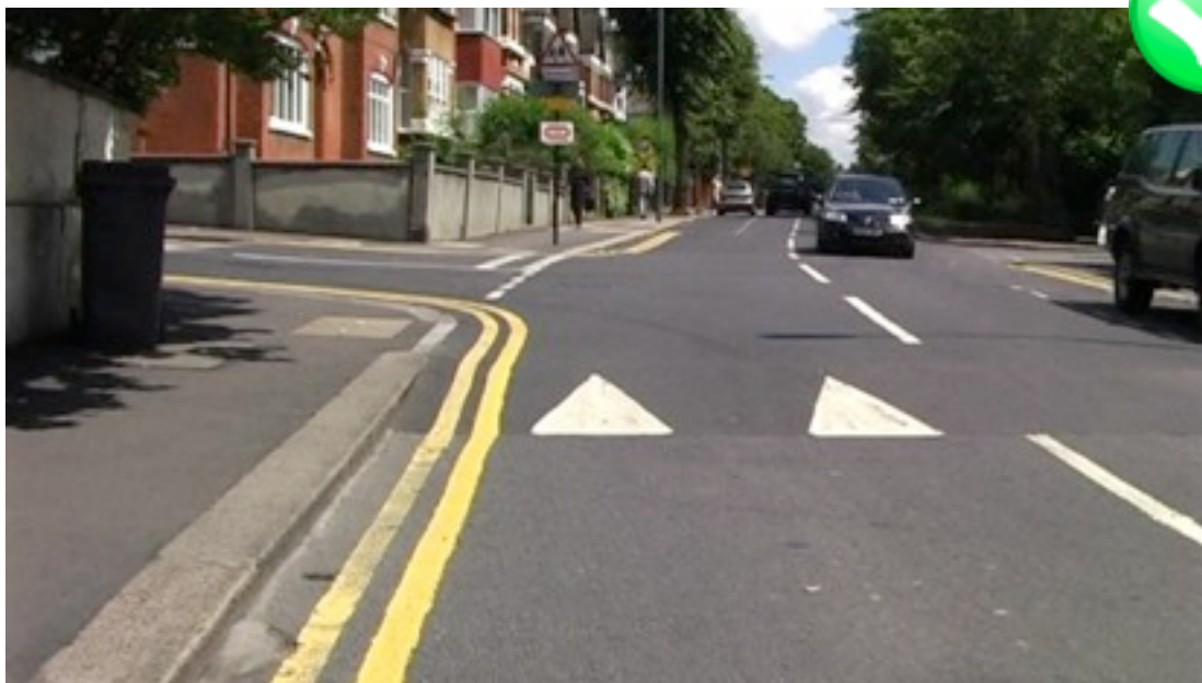
Cycle-positive measures don't necessarily need to include a cycle lane. This raised table on Church Hill forms part of an excellent scheme for cyclists, without any cycle lane. Other measures can control driver behaviour and traffic speed.
