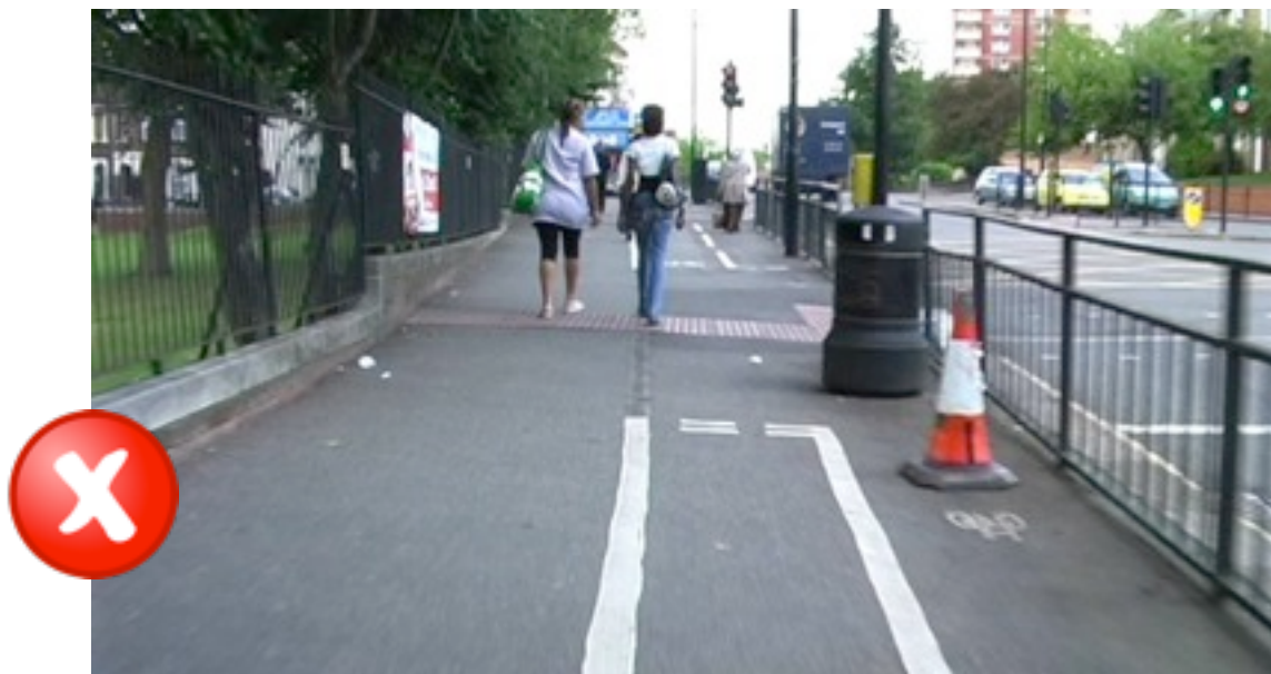
Obstacles (bin and cone) unnecessarily block part of this cycle path, which is also located on a busy pavement where pedestrians routinely walk into the path. Pavement cycle lanes often cause priority conflicts with drivers at crossings.
